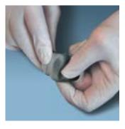
3. Apply to surface to be repaired within 2 minutes of mixing. Force into any cracks or holes and strike off excess material, preferably with a tool moistened with clean water.
